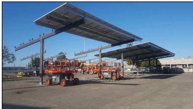
Figure 1- Solar Canopy Installation at WSP
