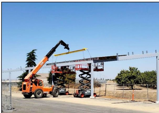
Figure 2 - Solar Parking Canopy Installation at CCWF
