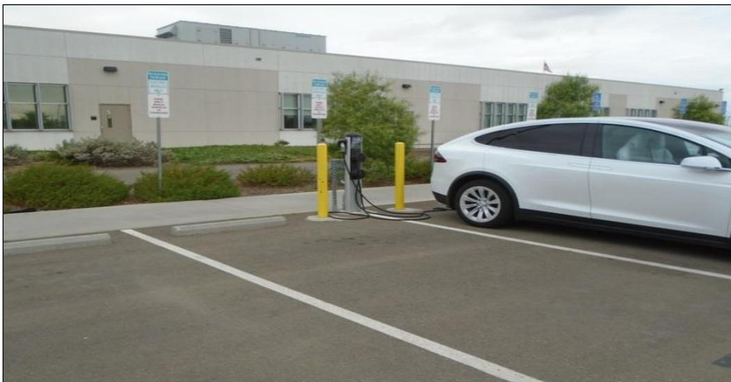
California State Prison, Lancaster (LAC) – During the construction of the Enhanced Outpatient Program Office and Treatment building, one Level 2 dual port charging station was installed to support workplace charging (activated 2014).
