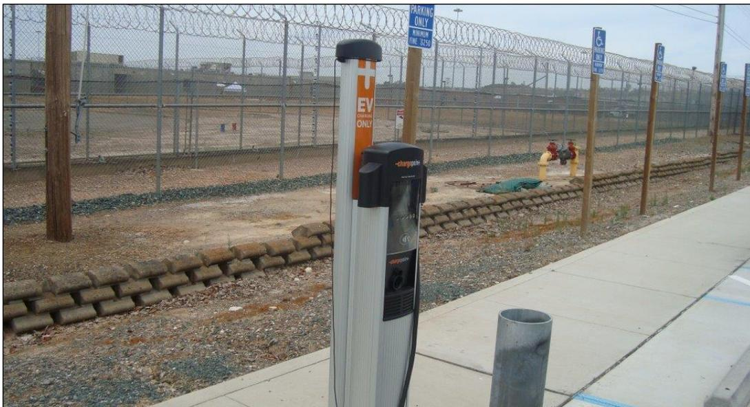
Richard J. Donovan Correctional Facility (RJD) – During the infill project at this site, five Level 2 dual-port charging stations were installed to support workplace and fleet charging (activated 2017).
